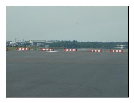
FIGURE 2 – A typical row of marker boards and lights, as placed at 260 m from the temporary runway end lights
