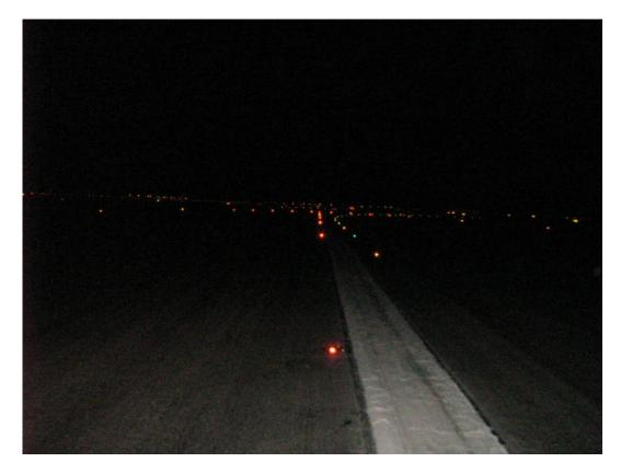
Figure 4. Distance-coded runway centre line lights and runway end lights near the shortened end of Runway 20C
