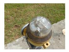
Figure 2. Approach light with broken top cover
