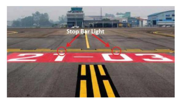
Figure 3: Stop bar lights at runway holding position
