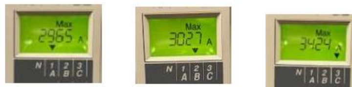
Fig 4 : Max Current at L1, L2, L3 of Bus Tie
