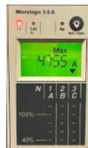
Fig 6 : Max Current at L1, L2, L3 of AFT PS ACB
