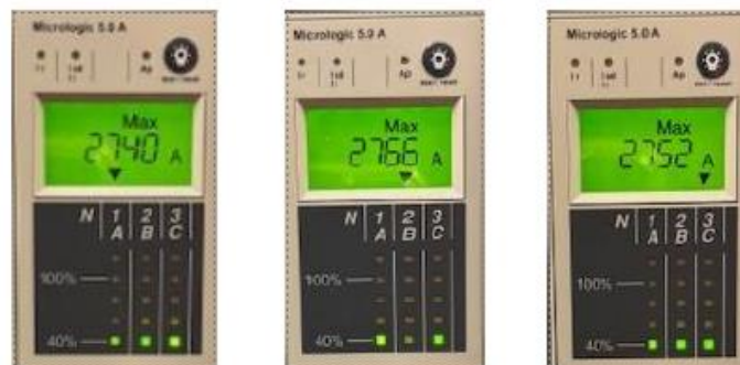
Fig 2 : Max Current at L1, L2, L3 of AFT PS ACB
