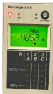
Fig 6 : Max Current at L1, L2, L3 of AFT PS ACB
