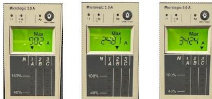
Fig 6 : Max Current at L1, L2, L3 of Bus Tie
