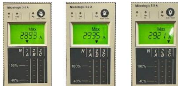
Fig 4 : Max Current at LT, L2, L3 of AFT SB ACB
