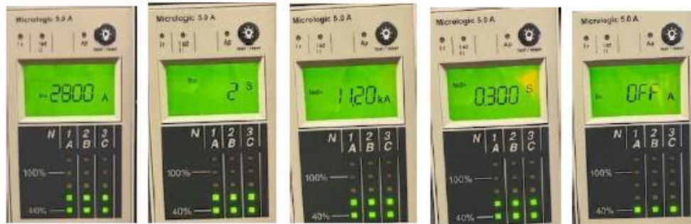
Fig 1 : Protection setting of Micrologic 5.0A at Incoming Feeder Aux Swbd AFT PS ACB
