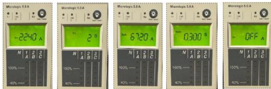
Fig 5 : Protection setting of Micrologic 5.0A at Bus Tie
