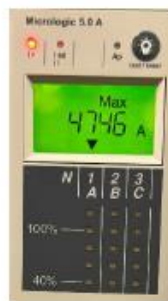
Fig 6 : Max Current at L1, L2, L3 of AFT PS ACB
