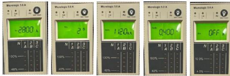
Fig 3 : Protection setting of Micrologic 5.0A at Incoming Feeder Aux Swbd AFT SB ACB
