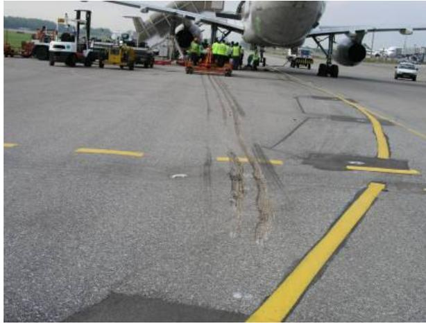
Figure 5: Gouging on Taxiway (about 50 metres)
