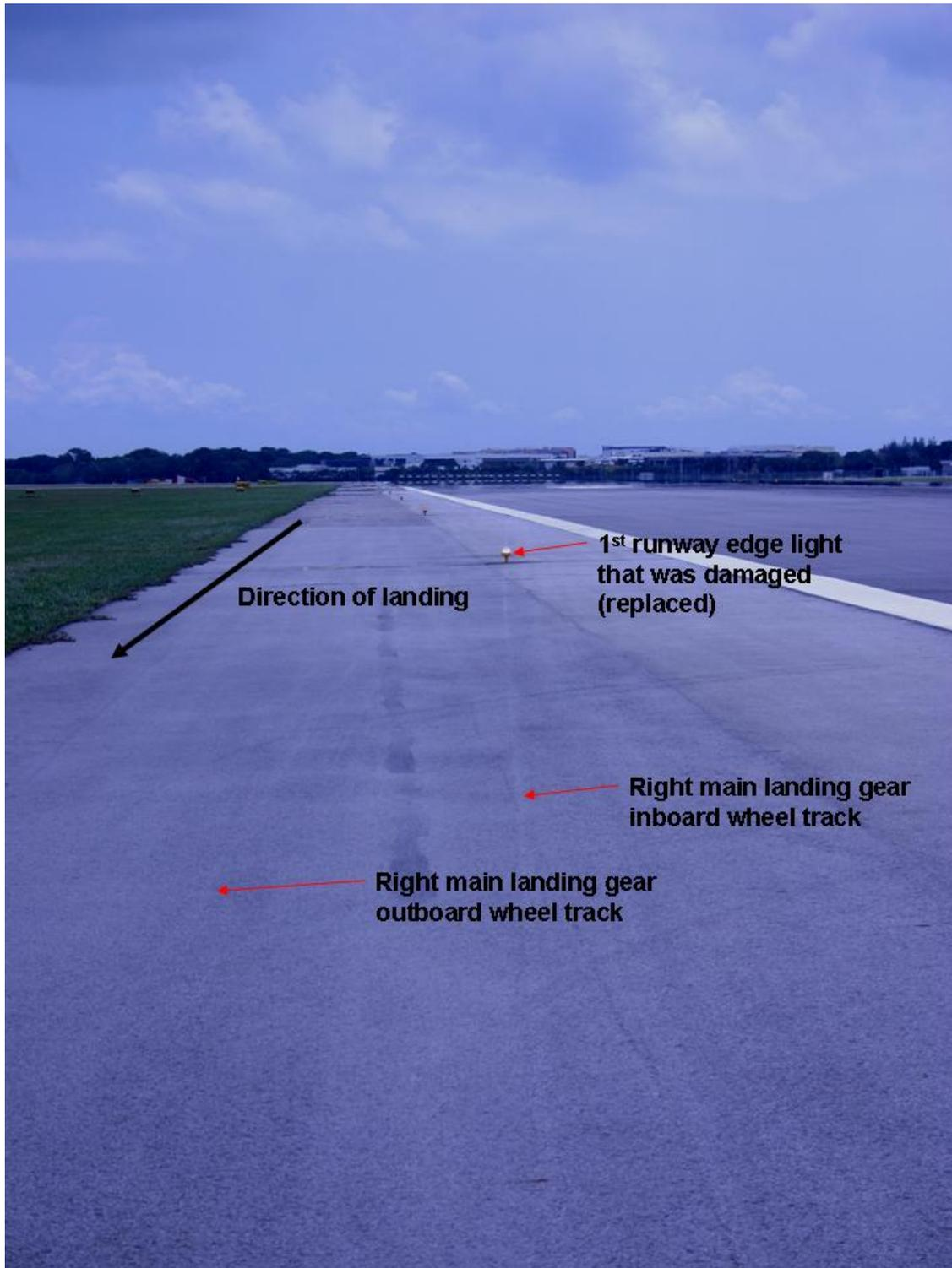
Figure 1: Wheel track of right main landing gear (looking against the direction of landing)
