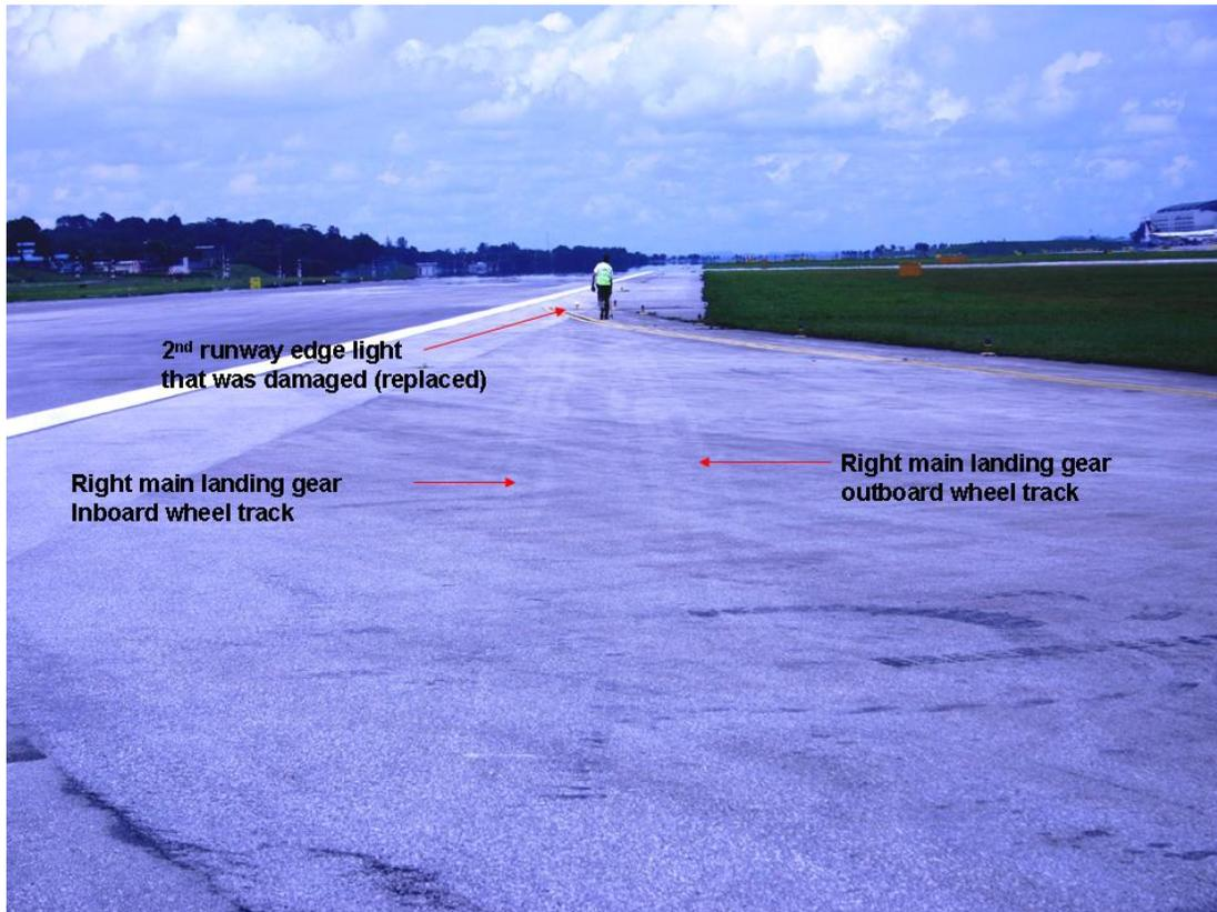
Figure 4: Wheel track of right landing gear on intersection of W7 Taxiway and runway (looking in the direction of landing)
