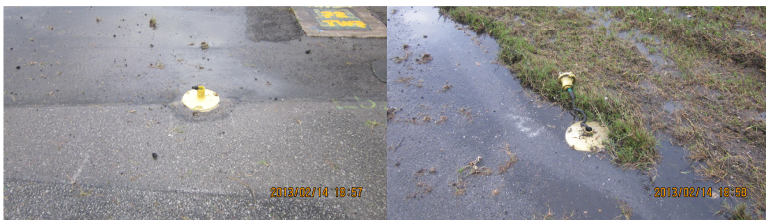
Figure 6: Damaged runway/taxiway lights
