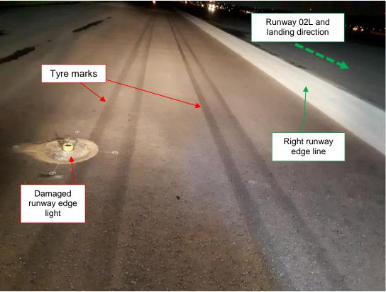
Figure 2. Damaged runway edge light and tyre marks
