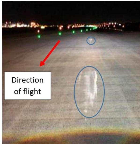
Figure 2: Scrape marks (circled in blue) on runway
