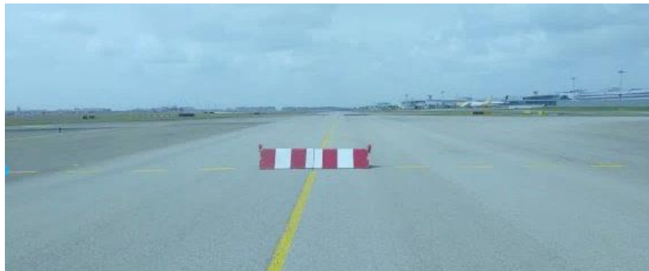
Figure 8: The marker board near the junction of Taxiways T and P2 before the incident
