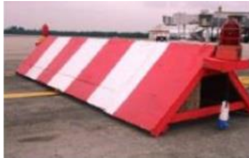
Figure 7: Typical marker board with an obstacle light on each end
