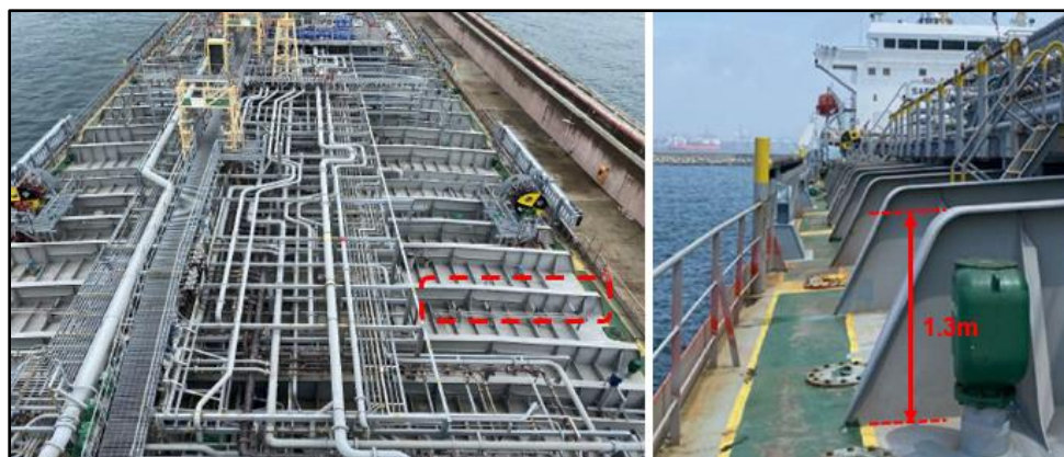
Figure 2 – View of the deck and raised deck frames (Source: the Company)
