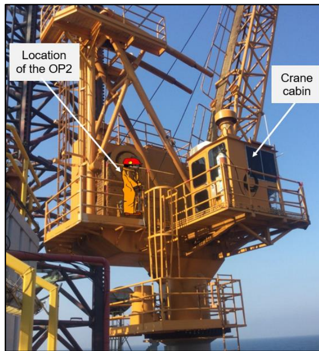
Figure 2 – location of the OP2 referencing to the crane cabin (Source: the Company)
