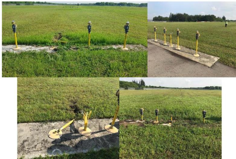
Figure 1. Damaged approach lights
