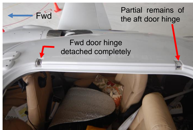
Figure 3. Damages on the hinges of the door
