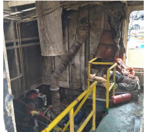
View of engine room and access door
