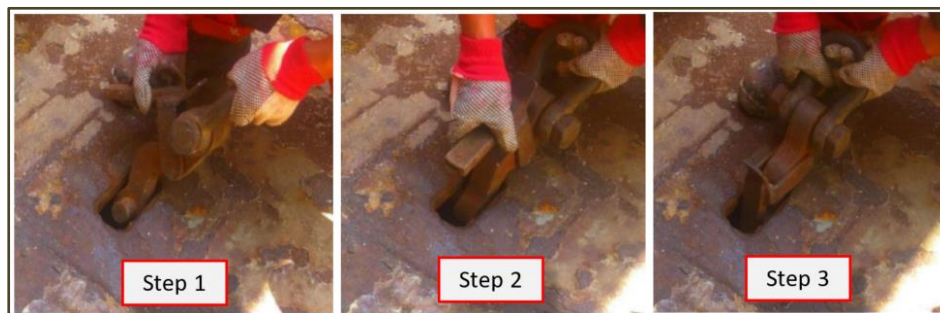
Figure 11b – Sequence of locking the lifting hook to the pontoon (Photo source: the ISM Manager)
