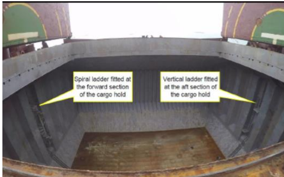
Fig. 1 - Cargo hold No.3 viewed from vessel's portside
