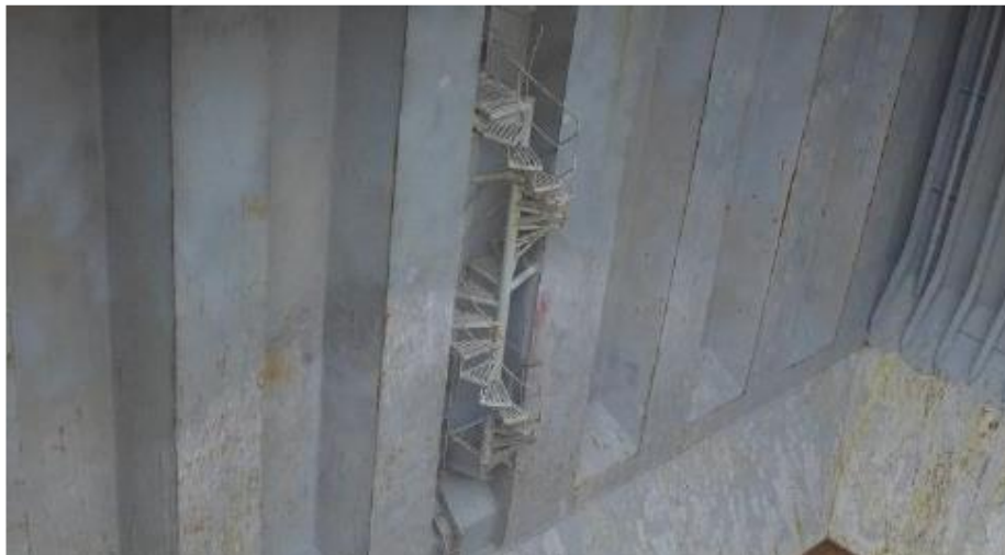
Fig. 5 - The forward access provided by spiral ladder
