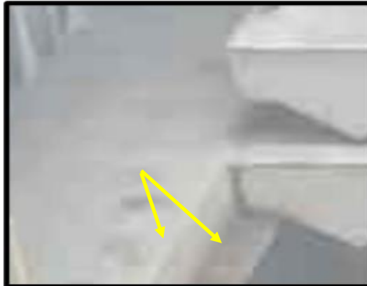
Figure 3: Zoomed in view of the walkway and edge showing similar colour - grey.
