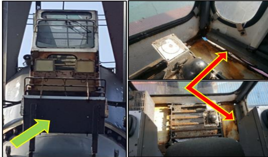
Figure 4b: External and internal photographs of crane no.2. Severe corrosion on the right-hand-side of the floor plate which had separated from the main cabin frame (red arrows). These photographs were taken after the rubber mats were removed and the area was de-rusted by the crew. Inspection platform (green arrow) – details in paragraph 1.5.6
