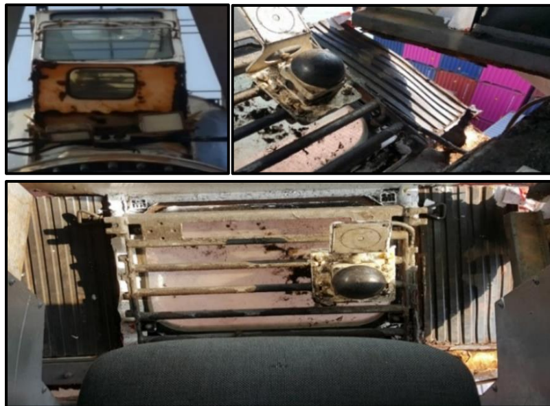
Figure 4c: External and internal photographs of crane no.3 cabin (clockwise from top-left) - the corroded condition of the floor plate, the sheared off right-side portion of the floor plate, and the plan view of the sheared floor plate
