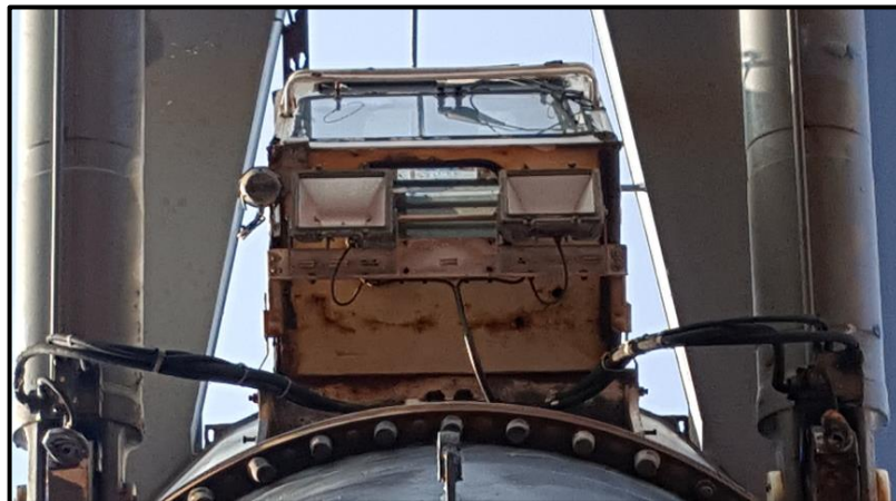
Figure 4a: Exterior of crane no.1 showing some corrosion on the floor plate
