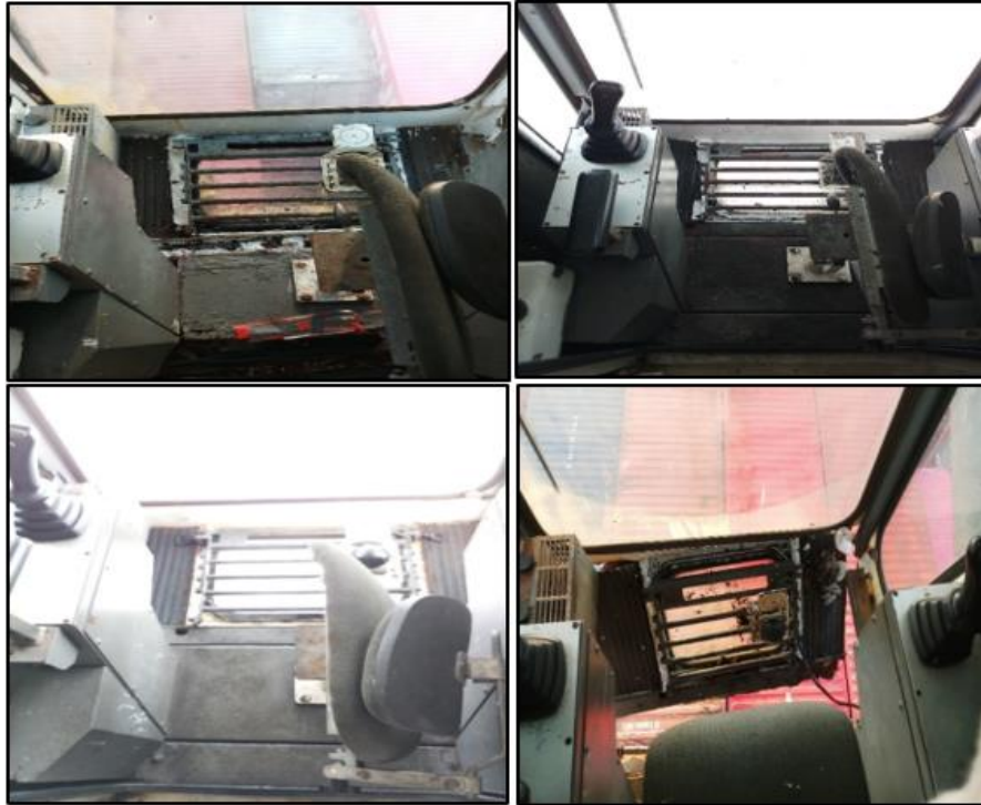
Figure 3: Condition of the floor plate taken from inside the cabin for each respective crane cabin. (clockwise from top left) – crane no.1, no.2, no.3 and no.4
