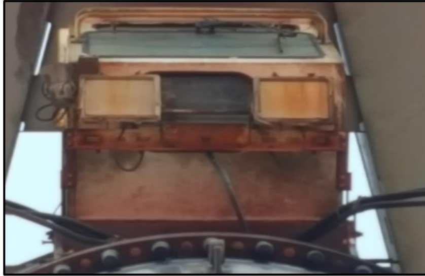
Figure 4d: External photograph of crane no.4 cabin displaying condition of the floor plate
