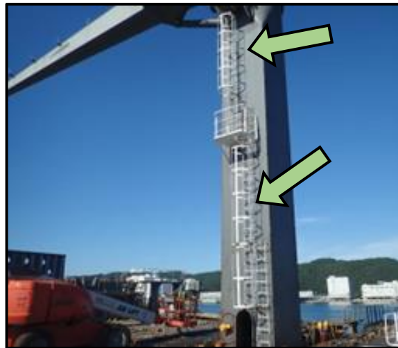
Figure 13: Fixed ladders installed on the cranes in a shipyard (green arrows).
