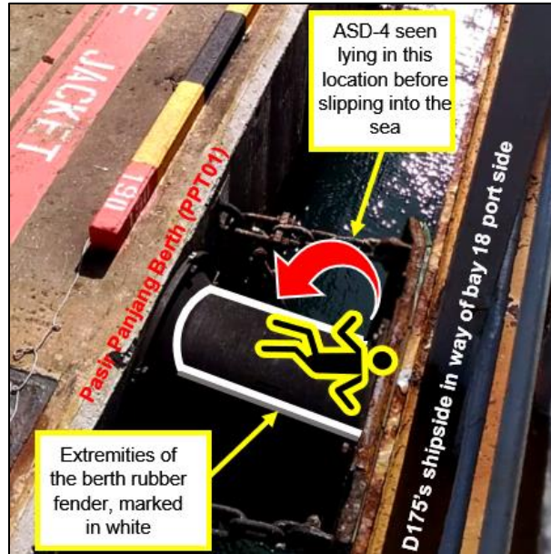
Figure 5 - Illustration showing the ASD-4's position after falling overboard before slipping into the sea as indicated by the direction of the red arrow ( Not to scale )
