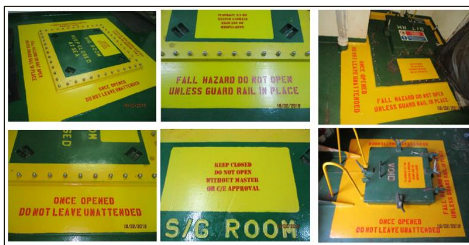
Figure 6 - Fall hazard warnings marked at various access openings (Photo source: the ISM Manager)
