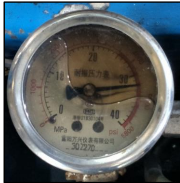
Figure 10 – Pressure reading on the air compressor gauge
