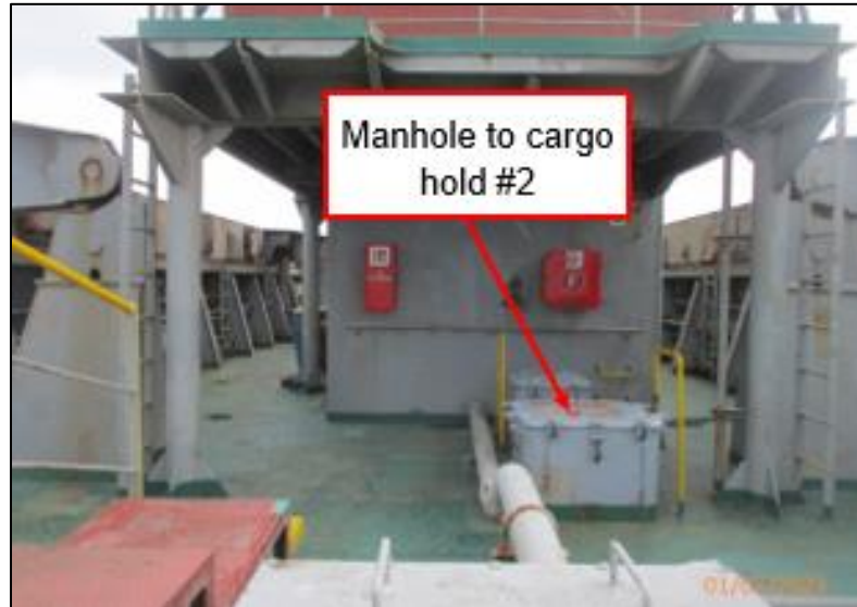
Figure 11 - Manhole to cargo hold #2 fitted with spiral ladder. Source: The Company. Annotation by TSIB.
