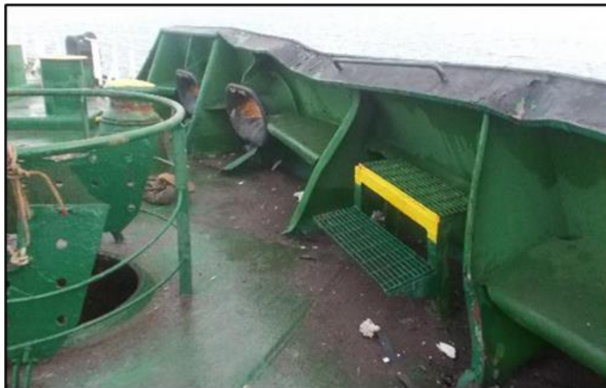
Figure 20 – Damaged section of the port side as viewed from the bow (Source: Company of AS)
