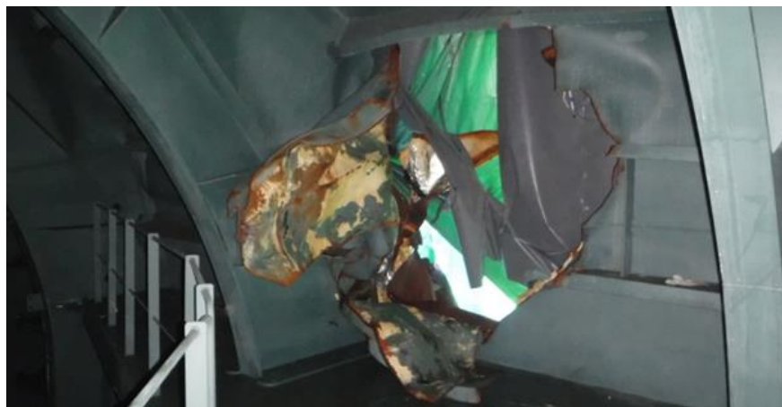
Figure 12 – Internal view of the vessel's damage (view from inside the tank)
