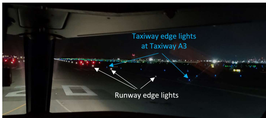
Figure 11: Taxiway edge lights, near the runway threshold, ON with runway edge lights ON
