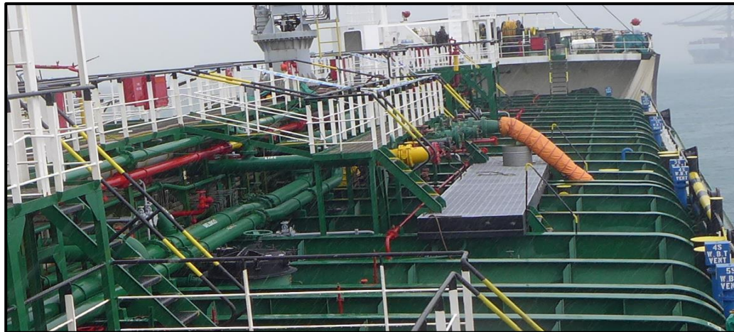
Figure 1a: One remaining chute connected to starboard manifold when investigation team was on board
