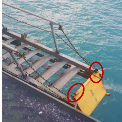
Figure 2 – Tilted bottom platform at the hinges and locations of locking pins (circled in red) – Annotations by TSIB
