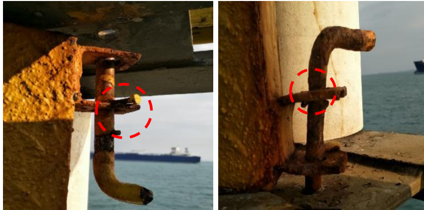
Figure 6 – Image on the left shows the outboard locking pin of the starboard accommodation ladder. Image on the right shows the inboard locking pin of the same ladder – Annotations by TSIB.
