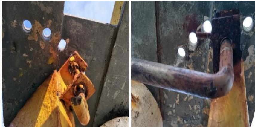
Figure 5 – Clockwise from top – Side view of port accommodation ladder, slots for inserting the locking pin (port side and starboard side) – Annotations by TSIB
