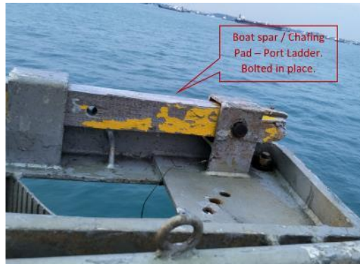
Figure 8 – Boat spar of the port side accommodation ladder bolted in place – Annotation by TSIB.
