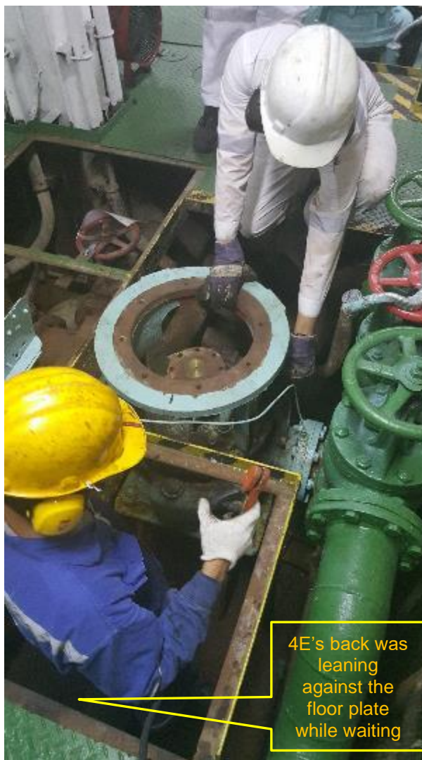
Fig. 3 – Illustration of 4E's approximate position at the start of welding work
