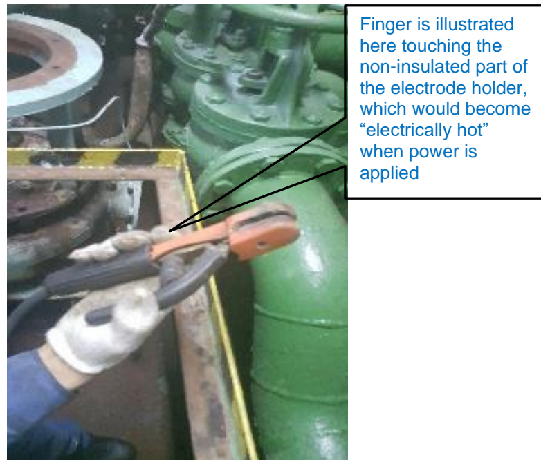
Fig. 4 – Illustration of how 4E was holding the electrode holder
