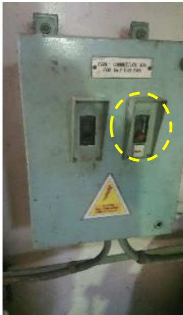
Fig. 10 - Power source in the engine room workshop
