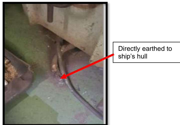
Fig.9 – Earthing of welding machine
