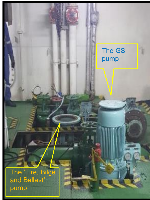
Fig.1 – FBB pump at engine room bottom platform
