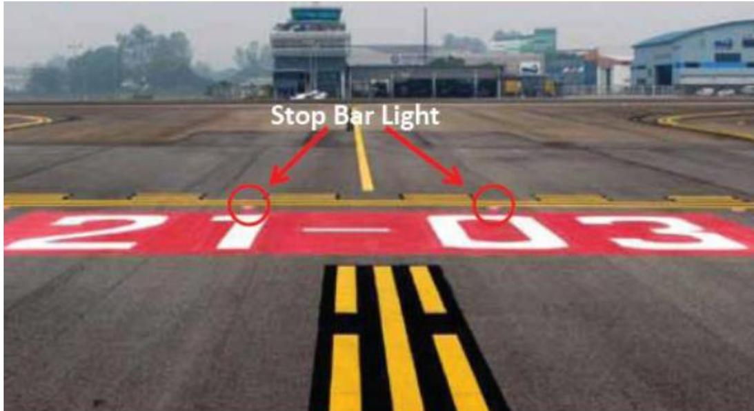
Figure 3: Stop bar lights at runway holding position
